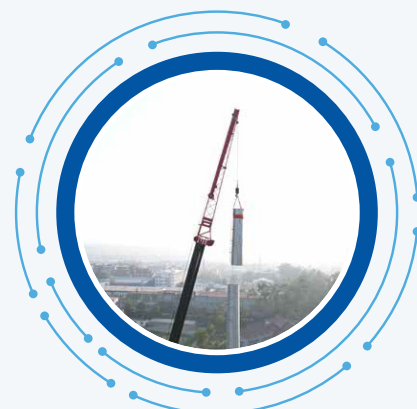
220 kV Double Circuit Monopole Installation - Dehradun, Uttarakhand
