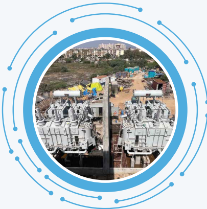
Underground Cable Network Project Himmatnagar & Idar, Gujarat
