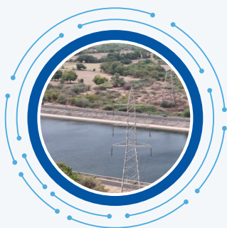
220 kV River Crossing Project (Government)
